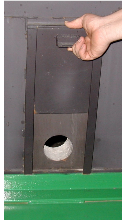
Access door for lighting
